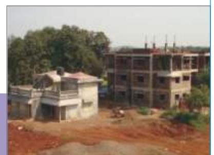
Principal & Staff Quarters (Under Construction)
