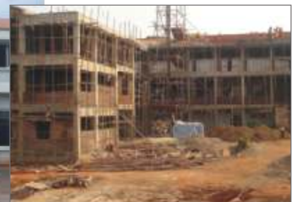
Institute Phase II under construction
